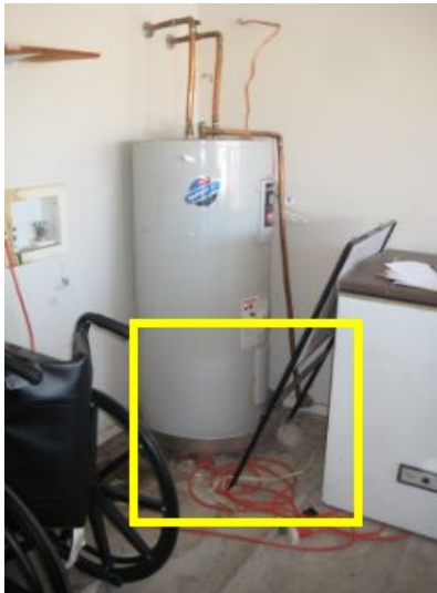
Unit is exposed to the elements
